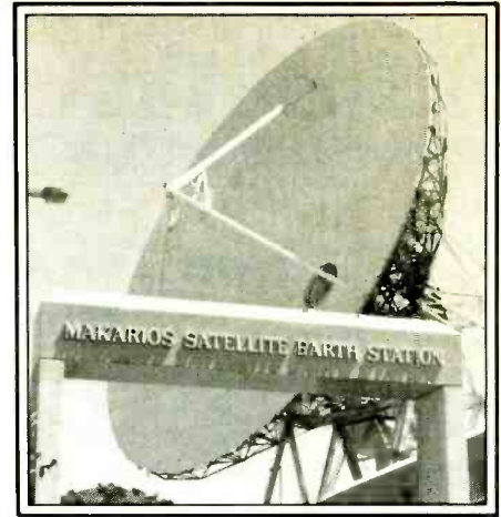
The Makarios Satellite Earth Station, on Cyprus, was a Class A Intelsat station that used a 30 meter dish with a forward gain of 62.84 dbm at 6 GHz. This station sent hostage-related TV coverage to the U.S. and Europe.
