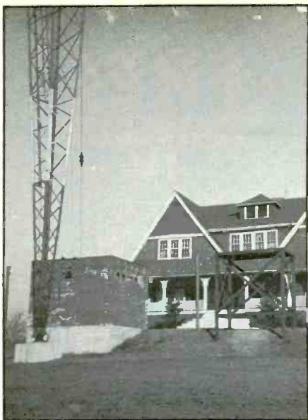
The WAAB/WNAC transmitter building, matching shack, and the lower part of the station's tower, circa 1936.
